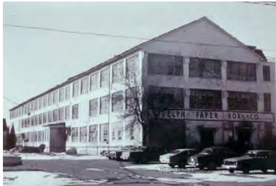
View of the heritage building from Huron Street in 1975 (Wellington County Museum & Archives, sl 07054)
