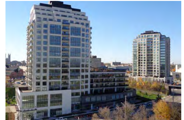
River Mill and RiverHouse
