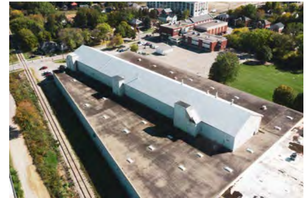
Aerial view looking southeast
